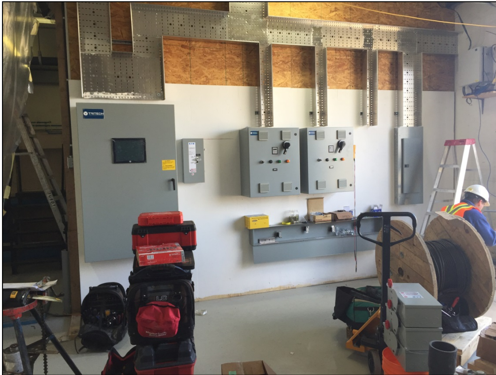
March 24, 2016: Electrical cable installation – electrical cable being pulled from control panels to various instrumentation and process equipment.
