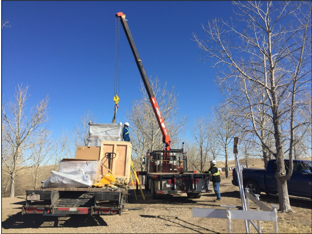
March 07, 2016: Filter Tank Delivery and Placement – filter tank delivered to the WTP site and set in place onto the epoxied housekeeping pad.
