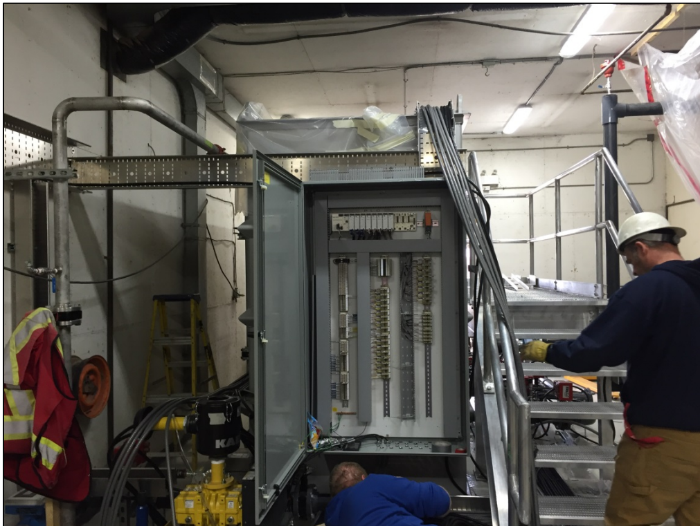
March 24, 2016: Electrical cable installation – electrical cable being pulled from control panels to various instrumentation and process equipment.
